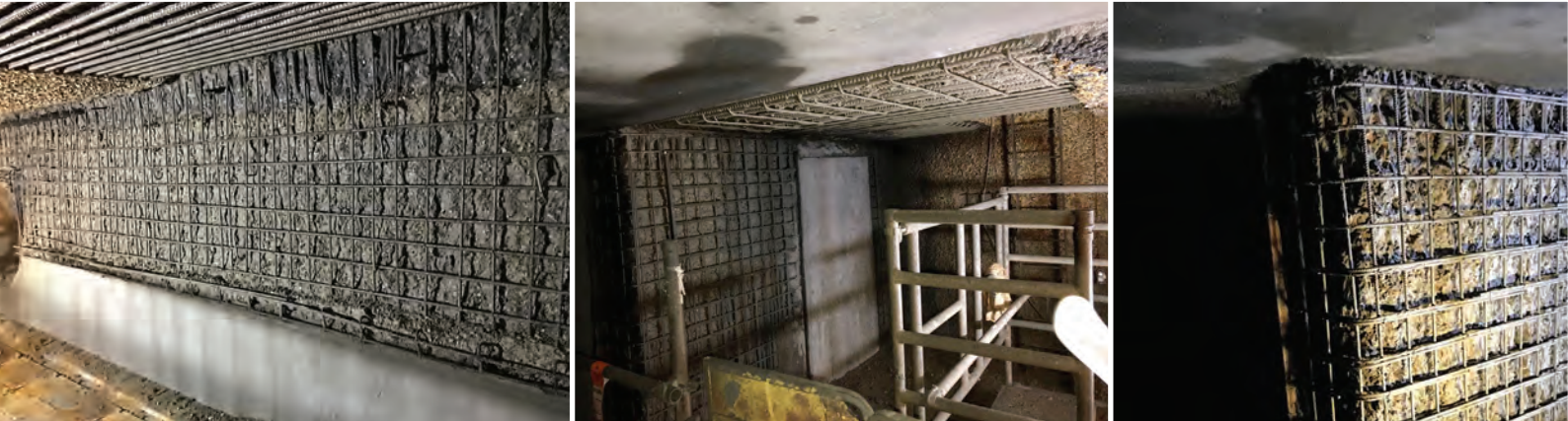
Hydro-demolition to remove defective concrete and expose and prepare the steel reinforcement.
