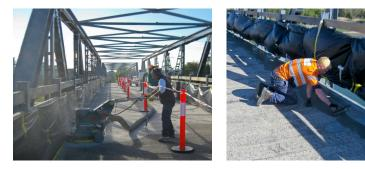
"The Intercrete 4852 system was chosen for its excellent abrasion resistance and fast return to service capabilities. The client required an aesthetically pleasing flooring system that could be applied and returned to service with minimal downtime so the public wasn't inconvenienced. Intercrete 4852 has achieved this brief along with providing a repair system with outstanding long term durability, which has exceeded the client expectations"
