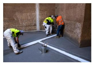
The specification demanded that the sealing system must have a 20-year minimum design life and be certified for contact with potable water to the Australian standard AS/NZS 4020. It was also important that the sealing system was flexible enough to accommodate movement of the wall and floor slabs and stresses associated with the ongoing use of the site, including daily partial depletion and filling and periodic emptying for maintenance.
