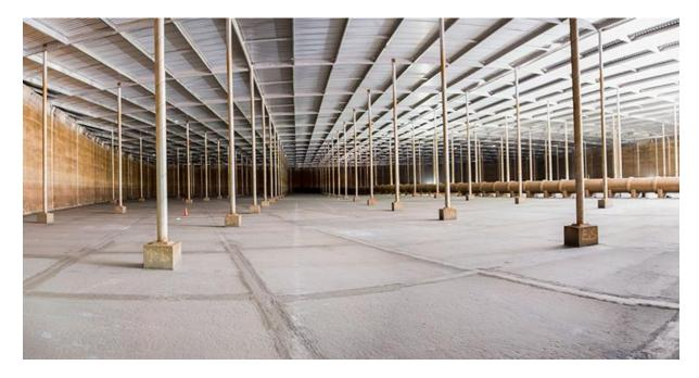
A major floor rehabilitation project has been carried out at an 86ML potable water reservoir in Australia. Over 73 tonnes of Intercrete® 4841 coating was delivered by air freight from the UK to Sydney for the refurbishment of Black Hill Reservoir in the Newcastle region of Australia.
