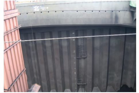
After 4 loadings of coal from high speed loading equipment
