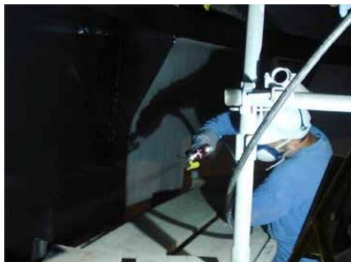
Interline 984C forms a smooth film which is easy to inspect, reducing inspection and repair time. Solvent free, thick film technology also allows a wide application tolerance, reducing the need for touch up and repairs.
